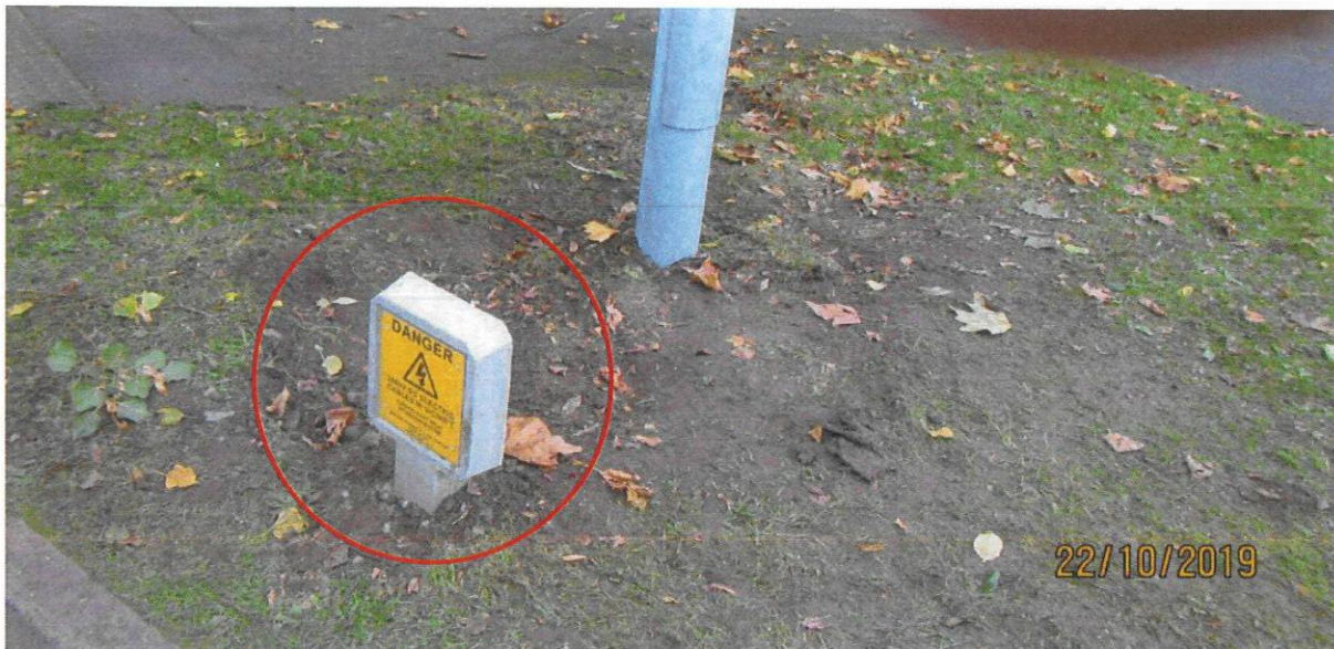
Figure 3.0 Safety marker post (circled red).
