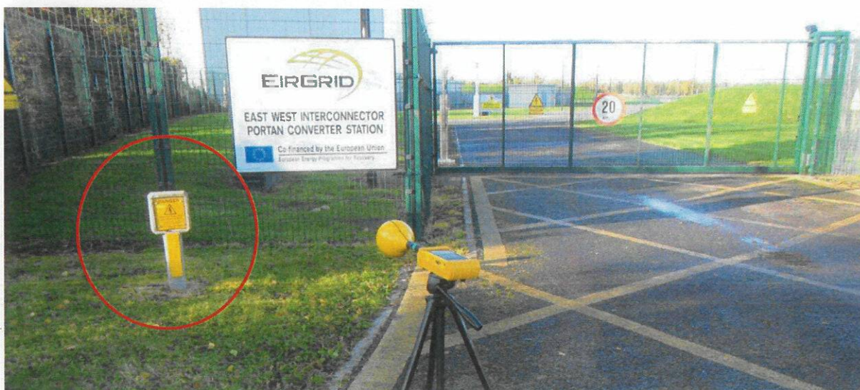
Figure 5.0 Safety marker post (circled red).
